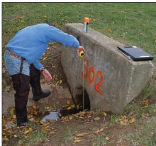
Figure 27: Measuring Outfall Diameter
