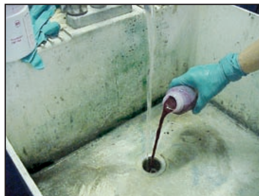
Figure 63: Dye Testing Plumbing (NEIWPCC, 2003)
